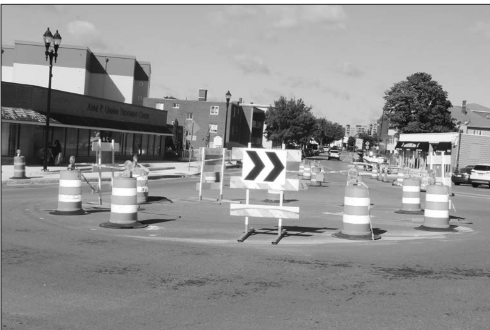
Orange and white barrels are in place as the intersection of Chelsea and Ferry Streets becomes the city's first roundabout which will reduce the wait times from the former traffic lights and improve the flow of traffic.
