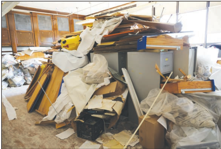
A former classroom is filled with discarded furniture, debris, and other materials awaiting removal.
