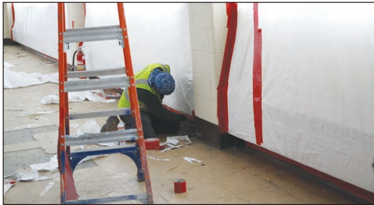
A contractor works inside the former Everett High School as environmental remediation continues throughout the building. #83) An abandoned science lab offers a glimpse into areas of the building that have sat vacant for nearly two decades.
