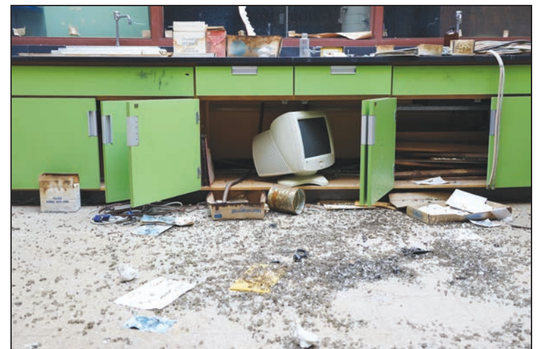
An abandoned science lab offers a glimpse into areas of the building that have sat vacant for nearly two decades.
